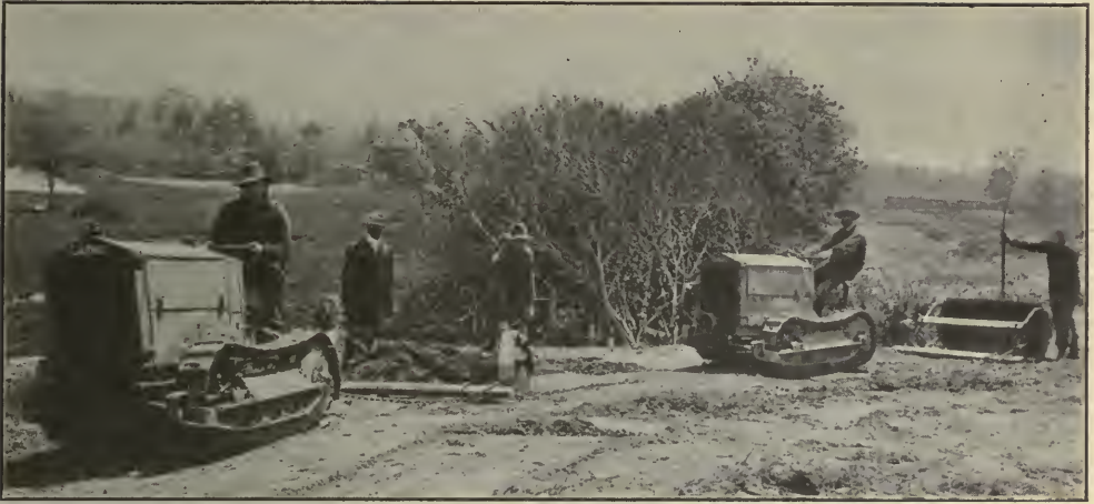
MEDIUM-WEIGHT TRACTORS HANDLING FRESNOS IN GRADING
